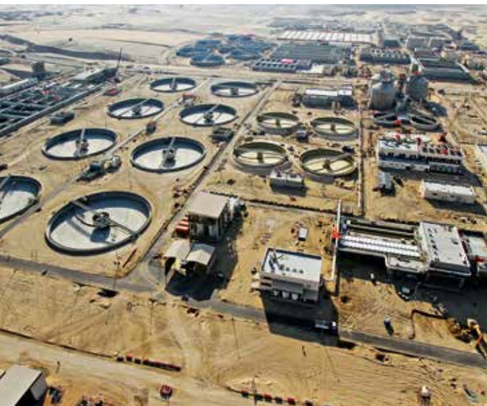
Al Wathba (afval)waterzuivering, Abu Dhabi, VAE
